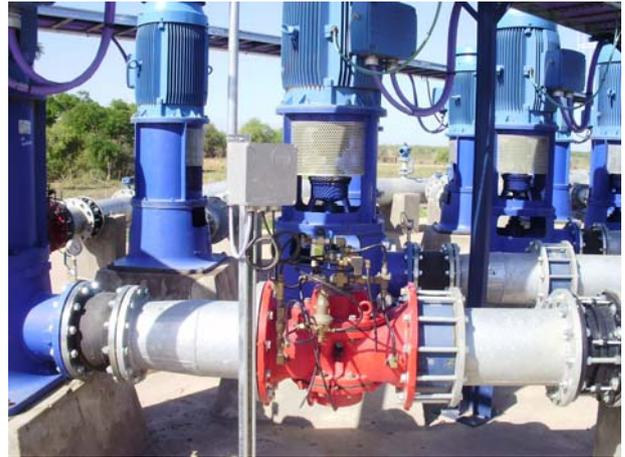
The 80 Valley pivots are equipped with ELECTRIC-OPENING PRESSURE-REDUCING VALVES, sized 8" \ 200mm Function code PR/EL.
