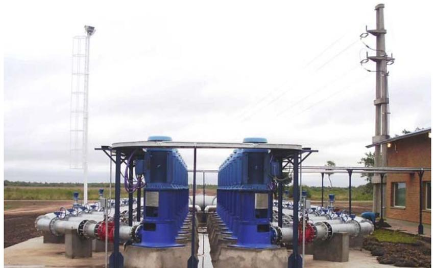
As known to all, in order to avoid risky water-hammer situations, the entire aqueduct must be filled in a controlled manner, so that the water is fed at a relatively low speed, slowly displacing the air in the pipe. To accomplish this, some of the pumps were equipped with pump-control and pressure-sustaining valves.
